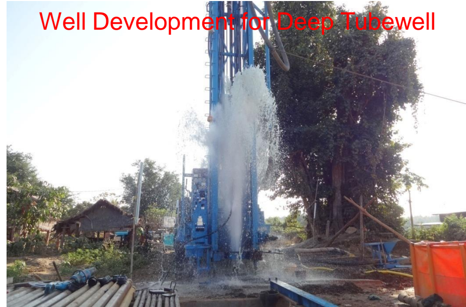
Well Development by Air Compressor
